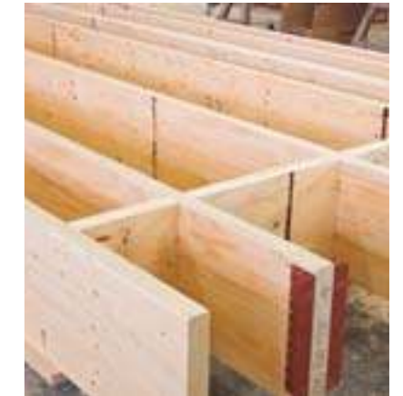
Pre-assembled box girders for roof construction.
