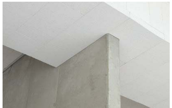
Lintel covering with wall connection
