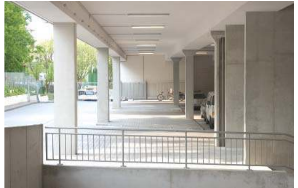
Ceiling insulation above entrance to large garage
