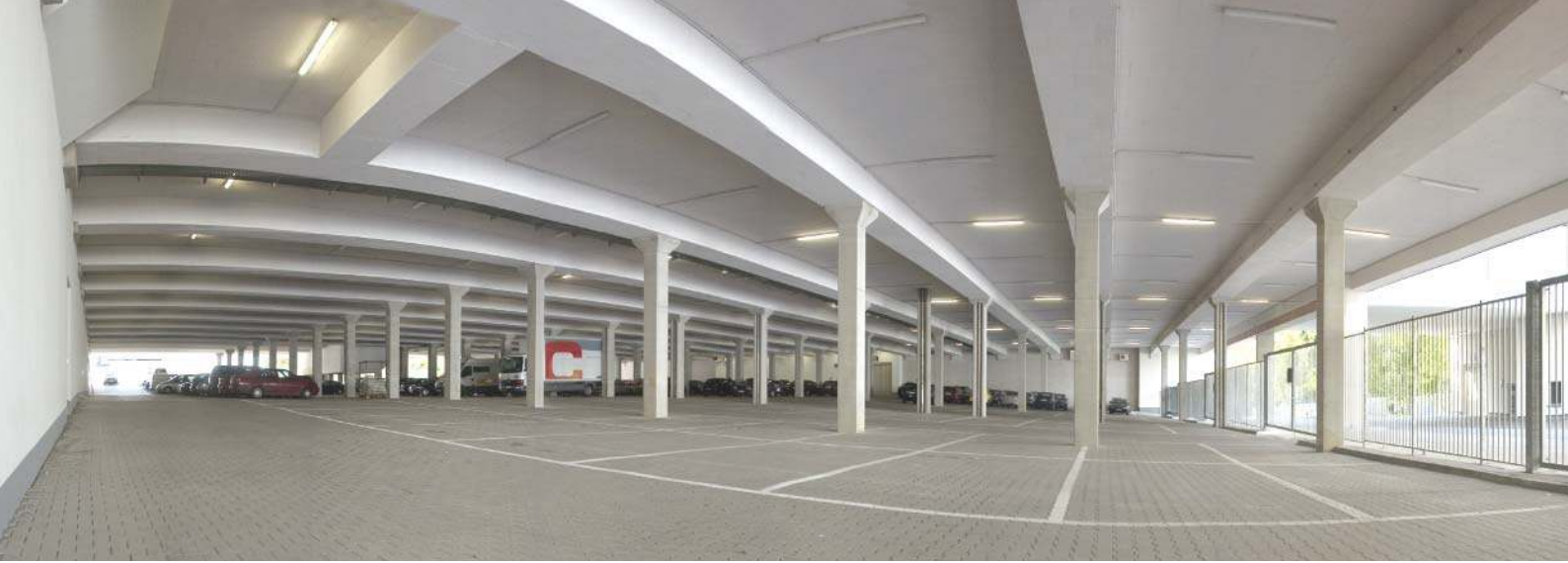
Large parking garage below Westphalia Hall B3 in Dortmund
