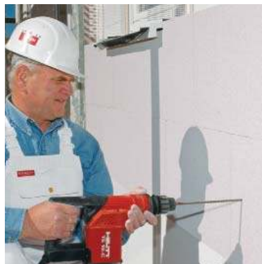
Ytong Multipor insulation boards must be fastened additionally with suitable anchors.
