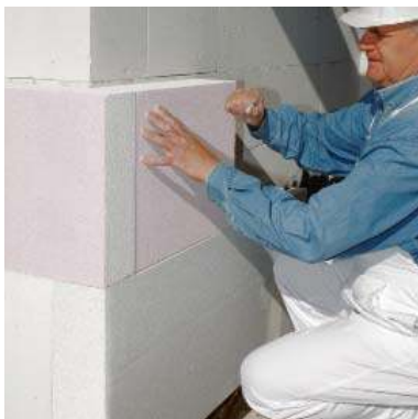
Press insulation board on to wall surface and slide against adjacent board.
