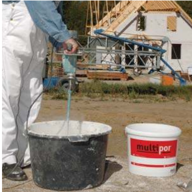
Mixing light mortar. 20 kg mixed with 8 l of water (mark on measuring bucket) yields approx. 30 l of adhesive mortar.
